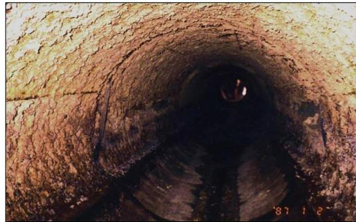
Figure 2: Severely corroded mushroom shaped
