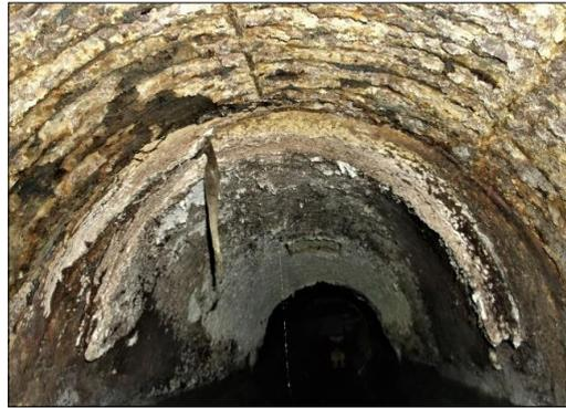
Figure 1: Corroded RCP (front) and FC (back)
