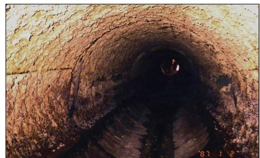
Figure 2: Severely corroded sewer
