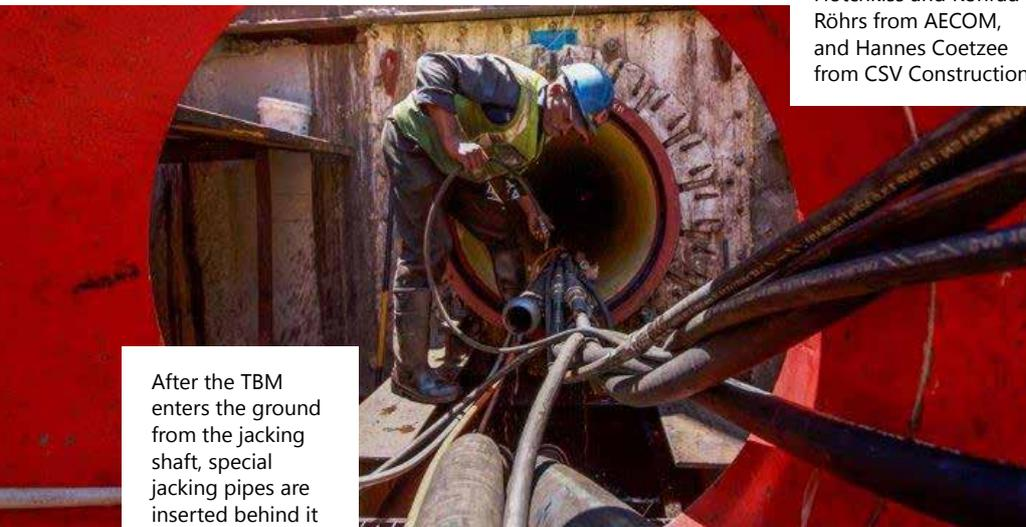
After the TBM enters the ground from the jacking shaft, special jacking pipes are inserted behind it
