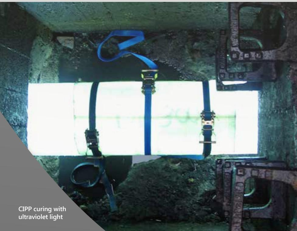
CIPP curing with ultraviolet light
