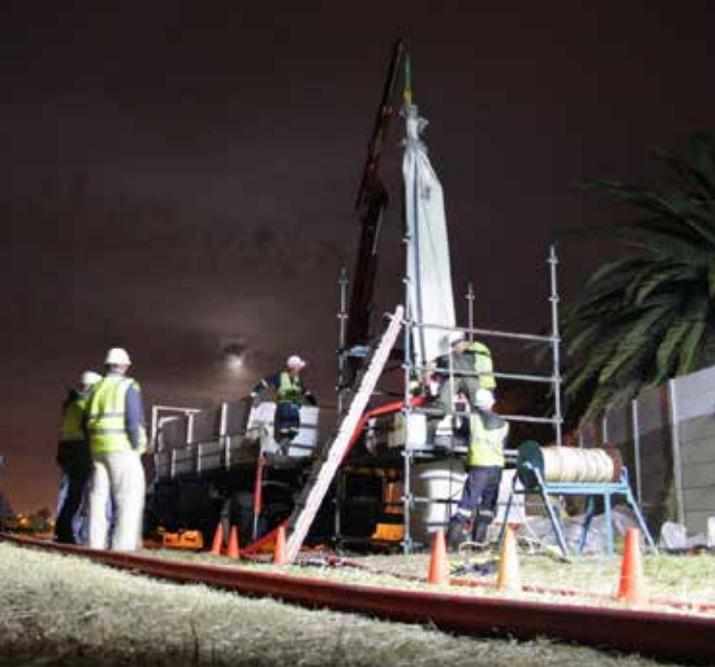
**ABOVE** Insertion of CIPP liner into the old 762 mm internal diameter Northern Areas Sewer (Photo: Timothy Hotchkiss)
