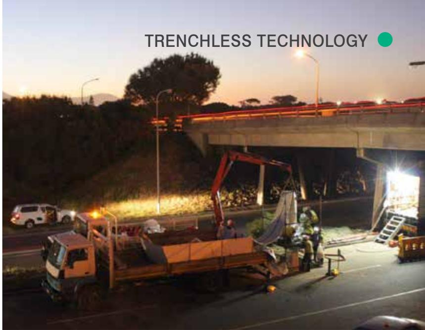
The company also installed a 35 m length of 160 mm diameter HDPE pipe by means of HDD in very close proximity to a residential boundary wall. Unforeseen rock material in the ground again provided a challenge. However, with the assistance of CSV Construction, this HDD was successfully completed without impacting on the nearby residents.
